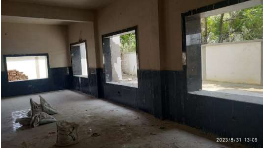
Auditorium/Multipurpose Hall Photograph -3
