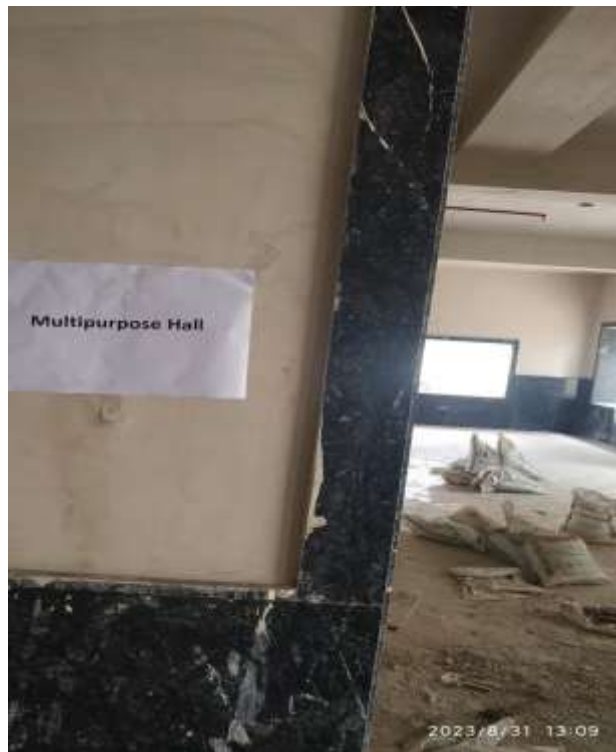
Auditorium / Multipurpose Photograph 2
